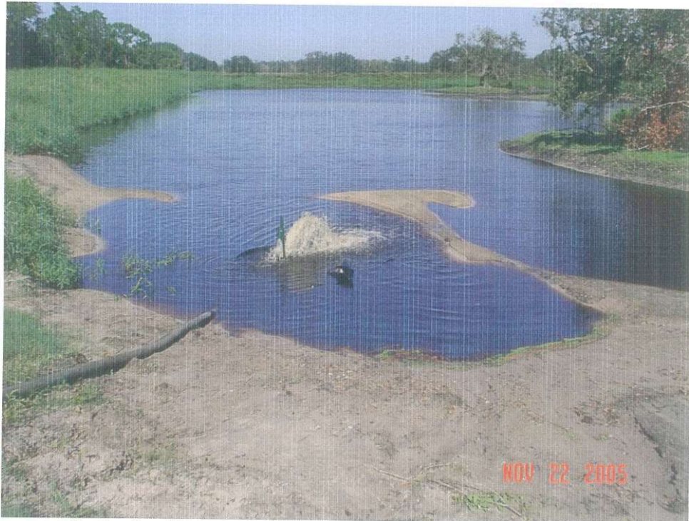
Photo 6 – Water at Pond Intake Discharging Upwards
