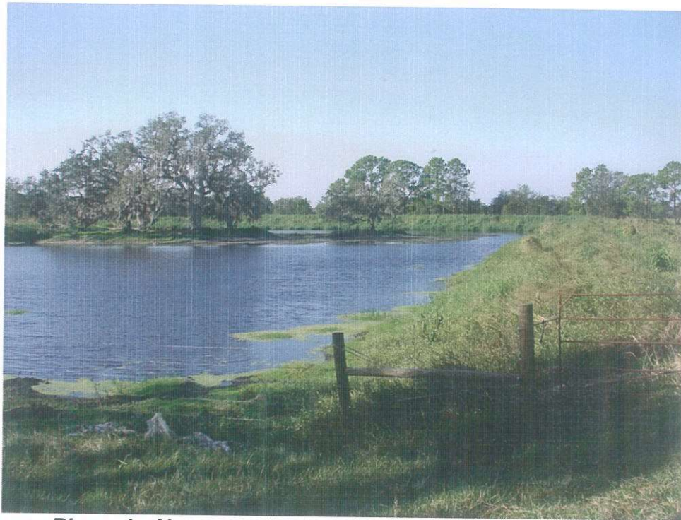
Photo 1 - North View of Settling Pond, from NE Corner
