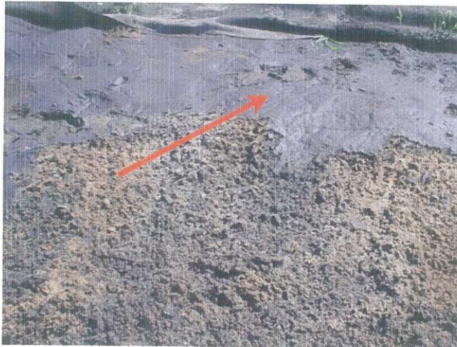
Photo 4 – Organic Silt Buildup on Humate Bed
