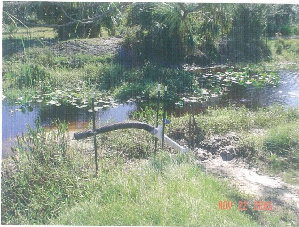
Photo 3 – Flexible Hose on Outlet from Humate Beds
