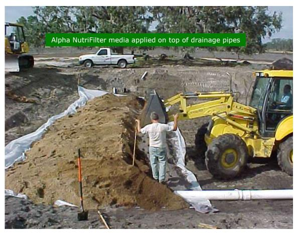
Alpha NutriFilter media is installed on top of the drainage pipes.
